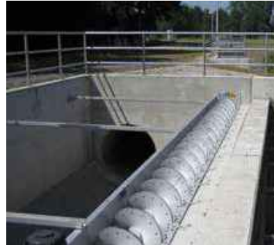
HUBER Storm Screen ROTAMAT® RoK1 installed on dry side of overflow weir.
