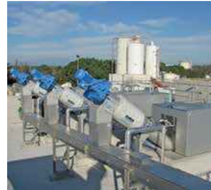
HUBER Perforated Plate Screen ROTAMAT® STAR protecting downstream membrane filtration systems.
