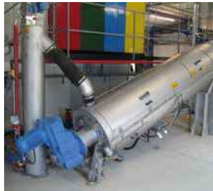
HUBER Screw Press S-PRESS: specific power consumption < 0.01 kWh/kg DR .
