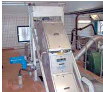
HUBER Fine Screen STEP SCREEN® SSF – the original STEP SCREEN®.
