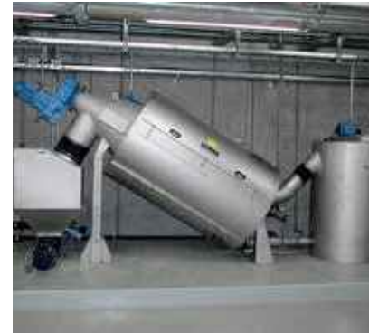
Extremely sturdy: HUBER Rotary Screw Thickener S-DRUM.
