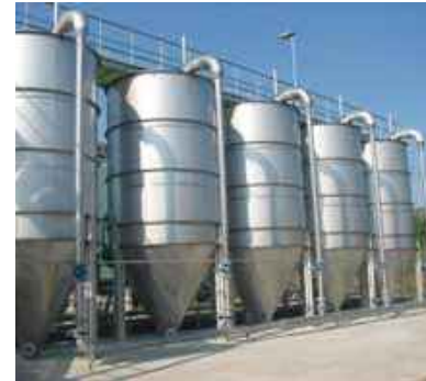
HUBER Sandfilter CONTIFLOW®, stainless steel design.
