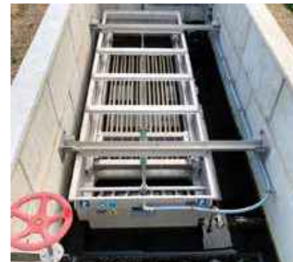
HUBER Heat Exchanger RoWin C installed in a concrete channel.
