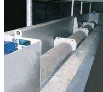
HUBER Storm Screen ROTAMAT® RoK2 installed on foul side of overflow weir.
