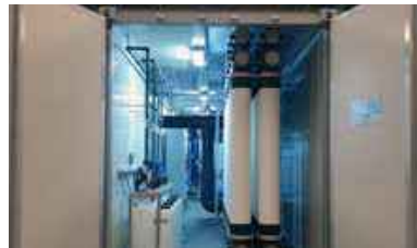
Pre-treatment stage using ultra filtration for suspensions removal.
