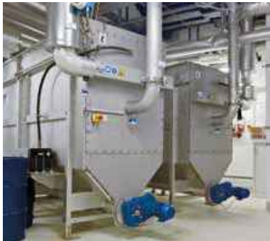
HUBER Heat Exchanger RoWin for energy recovery.
