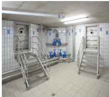
Pressure-tight HUBER doors for safe access to reservoirs.
