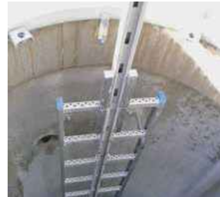
HUBER safety access ladder with fall protection.
