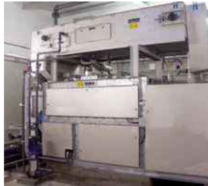
The HUBER Bogenpress B-PRESS can be combined with the HUBER Belt Thickener DrainBelt unit to further increase capacity.
