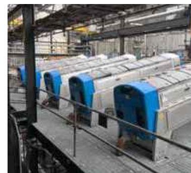
Sludge dewatering with HUBER Screw Press Q-PRESS® 800.2.
