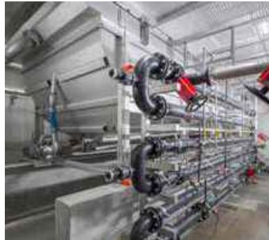
Dissolved Air Flotation Plant for reliable wastewater treatment.
