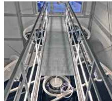
HUBER Active Carbon Filter CONTIFLOW® GAK, stainless steel design, for the removal of trace substances.
