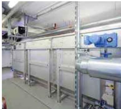
RoWin Heat Exchanger for energy recovery.
