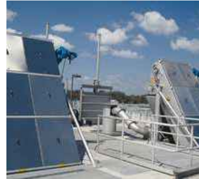
HUBER Belt Screen EscaMax® – versatile headworks screen with high separation efficiency.
