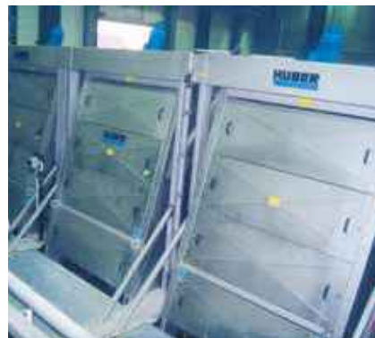
HUBER Fine Screen STEP SCREEN® SSV – the improved STEP SCREEN®.
