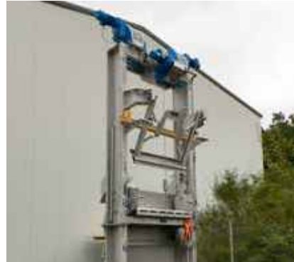
HUBER Grab Screen TrashLift for coarse material removal.
